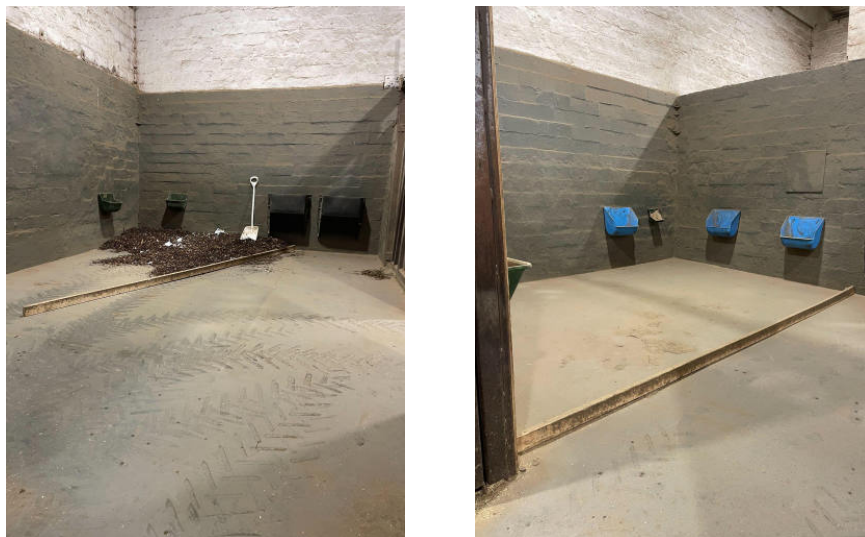
Picture 9 & 10. The enclosure on the day of conversion.
